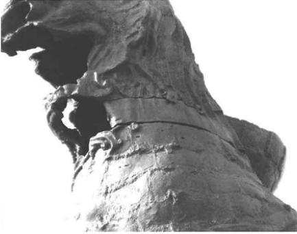
Figure 18. The Cangzhou Lion photographed in 1987. Note the modern repair and the missing lower jaw (photo by author).
