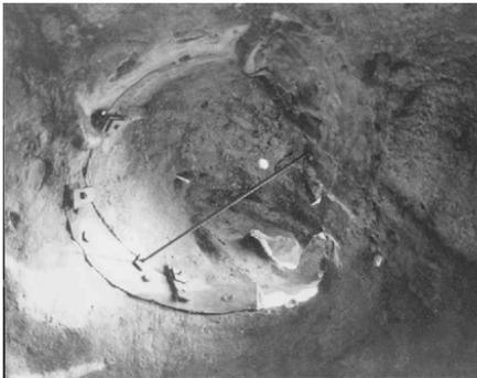
Figure 19. Inside the head of the Cangzhou Lion, showing more of the modern repairs. Part of the cast-in wrought iron reinforcement can also be seen extending from the center of the photograph to the lower right corner (photo by author).
