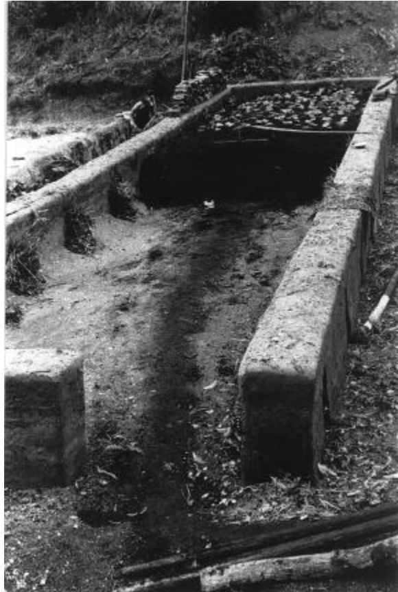
Figure 4. Stall furnace for crucible smelting of iron, partly loaded with crucibles packed in coal. Photograph by Dr. Knapp, 1936, in the archive of the Needham Research Institute, Cambridge; originally supplied to Dr. Needham by H. Dickmann in 1958. Dr. Dickmann states that the photograph was taken at “Kan Kong, 20 km east of Ping Huang, Hunan”; if this is correct it is the only indication we have that the crucible smelting method was ever used in Hunan.
