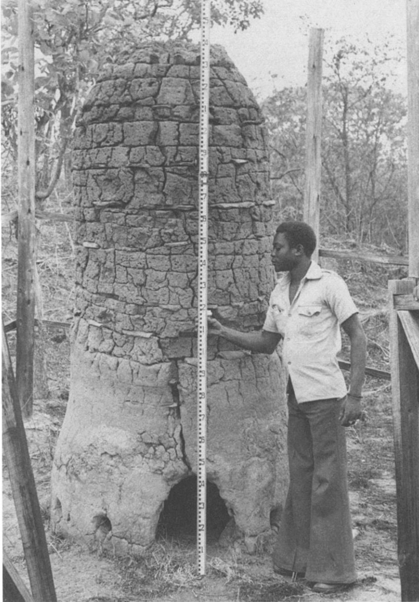
FIG. 3.—Bloomery furnace near Kasungu, Malawi. The stack is made of baked clay taken from termite mounds and is sufficiently high to permit the furnace to attain smelting temperature by natural draft rather than with an air blast provided by pumping bellows. The small holes around the base are for the insertion of tuyeres; the bloom was removed through the large opening when smelting was finished. The flat plates inserted in the upper part of the furnace are broken pieces of old tuyeres.
