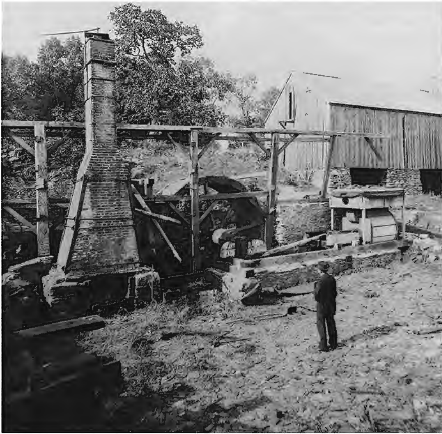
Fig. 12. This photograph of Windham forge in New Jersey was taken in 1892, about ten years after the forge was abandoned. The blowing engine, with its horizontal cylinder, is on the right. There is an accumulator for maintaining a steady blast pressure on top of the cylinder. The water wheel that drove the blowing engine is in the back. Remains of the bloomery hearth can be seen at the base of the brick stack, which encased the iron pipes of the heat exchanger that preheated the air blast. The remains of the forge hammer and the stamp mill used to pulverize the ore are not visible in this view. (Photograph courtesy George Sellmer)
