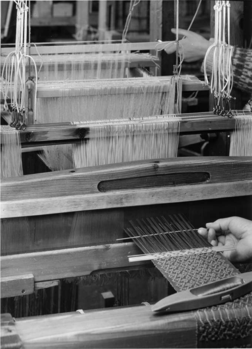
Figure 64 The rod for the ground pattern weft is left down, only the rod for the red pile warp is still lifted, and the knitting needle is put in before the next tabby weft can be woven.
