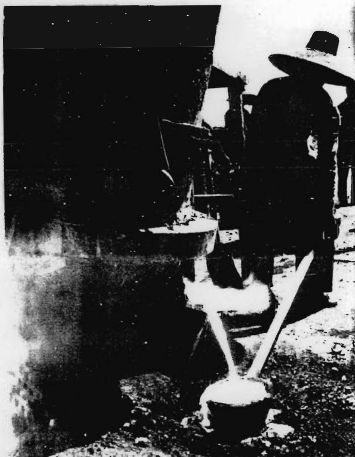
Small blast furnaces like this with a daily output of a ton go a long way towards pushing up the country's output of iron
